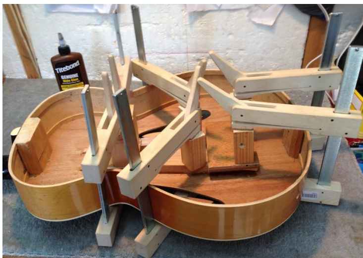
Photos 11 & 12: With the back off it was possible to assess the damage to the braces. One of them just had a failure of the glued joint but the other had partially ripped the surrounding surface. Both relatively easy to resolve.
