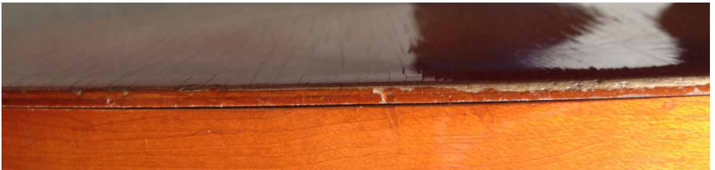
Photo 2: The back was pulling loose most of the way around the body.
